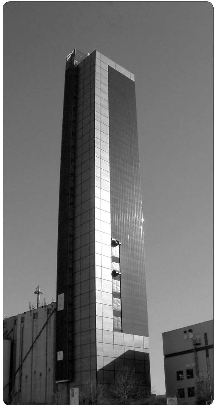
The Schapfen Mill Tower is a flour mill in Germany. The southern facade is faced with 1,300 CIS solar modules.
